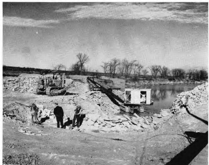
Between two workmen, Dave Kirby, official measurer of Fleet 188, watches the start of the cut to be made in solid rock 30 ft. wide, 10 ft. deep and approximately 75 ft. long.
